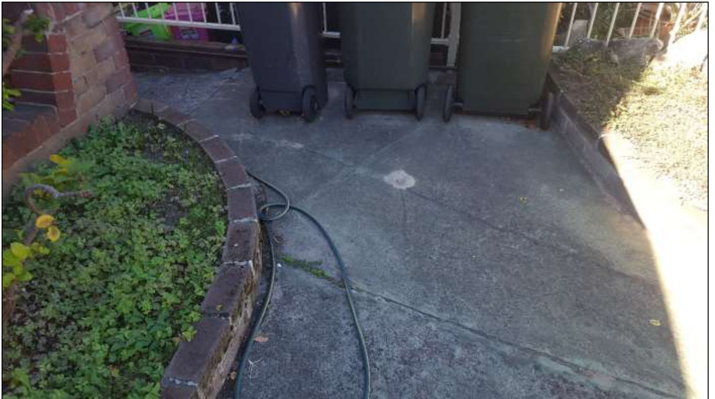
Minor Cracking of Pathway
