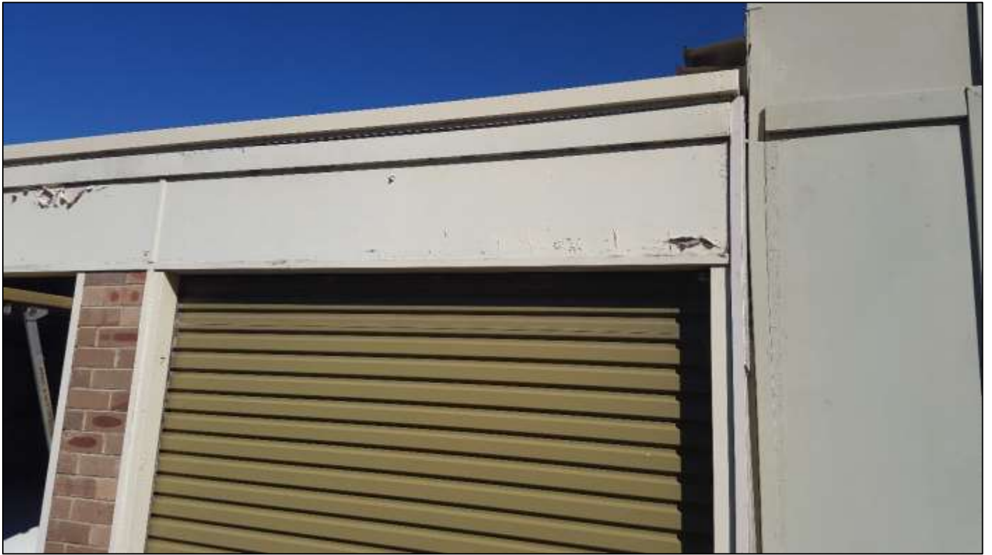
Potential ACM in Structure
