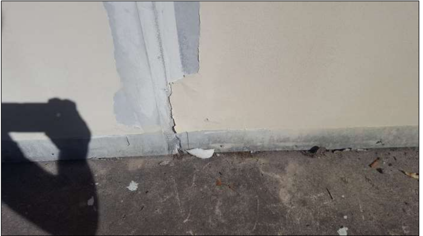
Potential ACM in Structure
