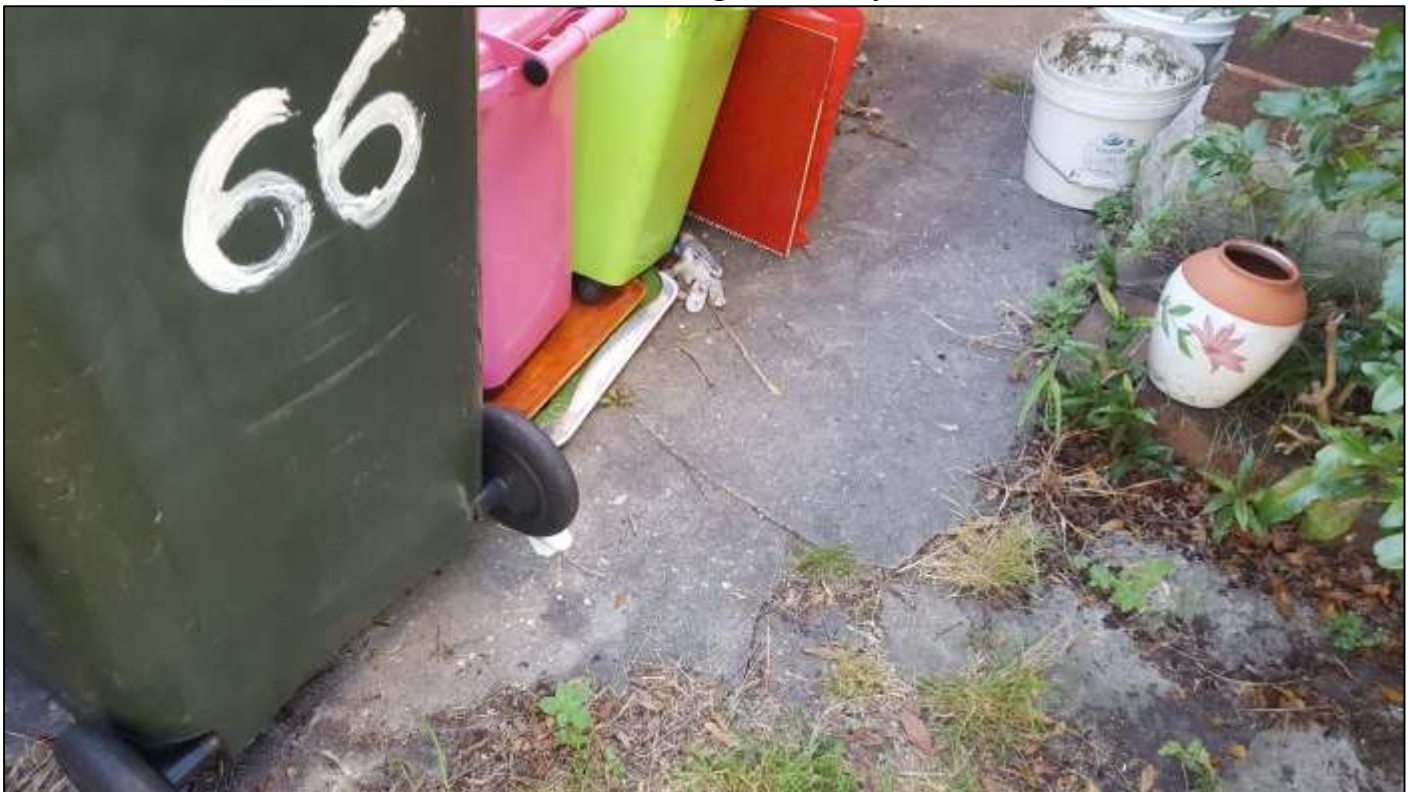
Minor Cracking of Pathway
