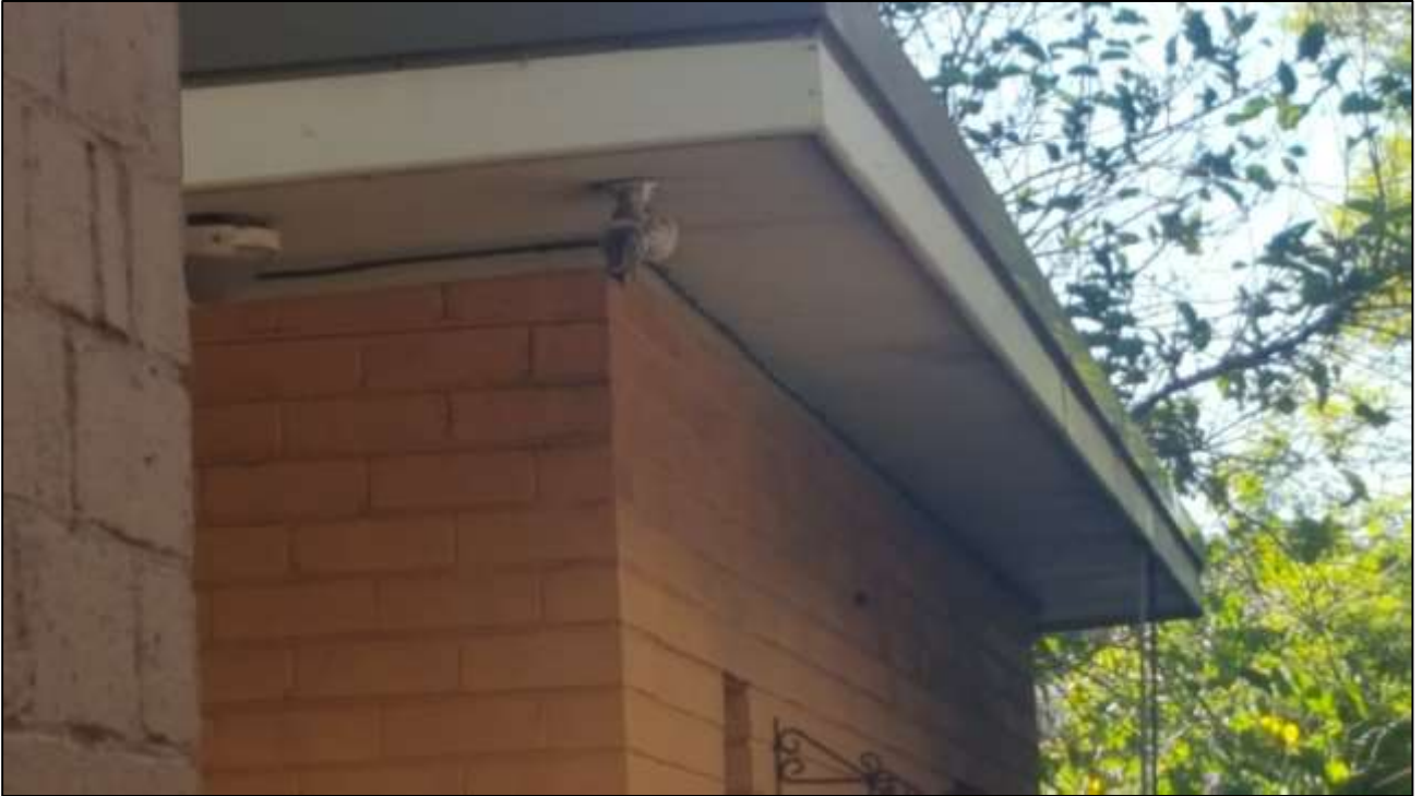
Potential ACM in Structure
