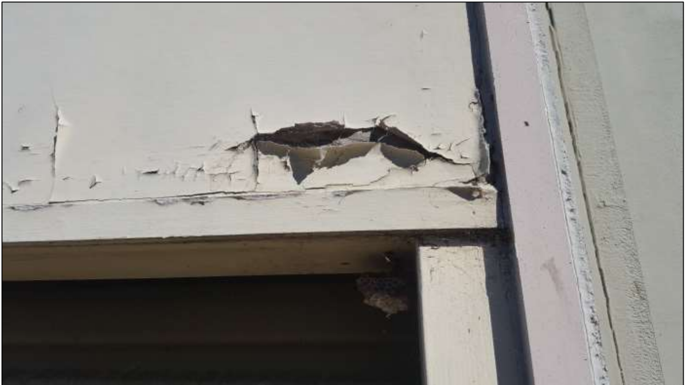
Potential ACM in Structure
